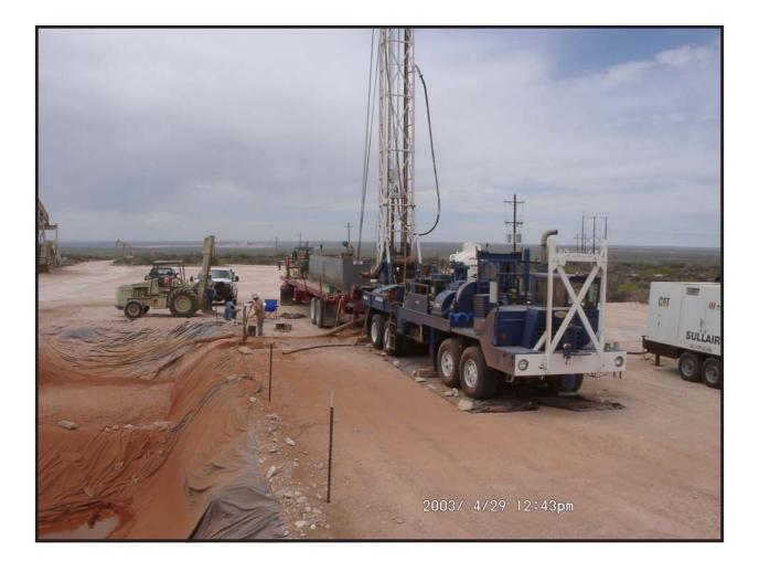
West Texas Water Well Service Rig #15 (Gardner-Denver 1500) on-site at SNL-2, viewed toward the west. The drill rig is set up for drilling with compressed air and foam, which is discharging into the mud pit to the left. IMC Kalium potash mine surface facilities and tailings are visible near the horizon (left center) over the front-end loader.
